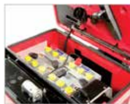
4 x 6v-180ah (5h) batteries
